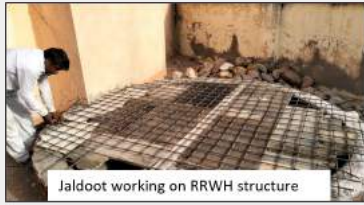
Jaldoot working on RRWH structure
