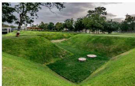
Figure 5: Rainwater recharge for flood mitigation at Torrent Pharmaceuticals Campus
