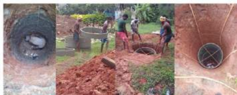
Digging of recharge wells. Source: Biome Environmental
